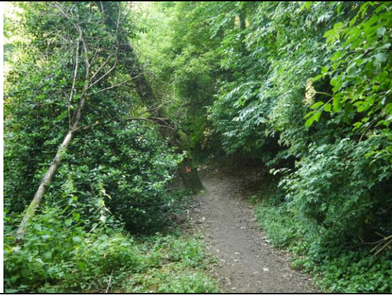
32. Subsidence on the wooded slopes
