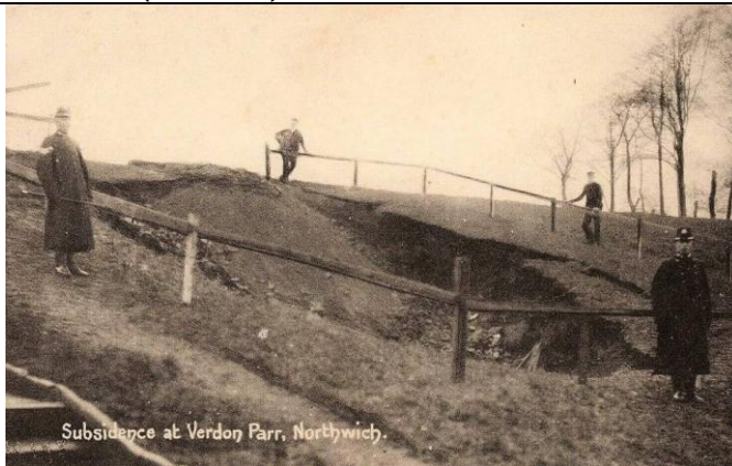
16. Subsidence on the slopes of Verdin Park
