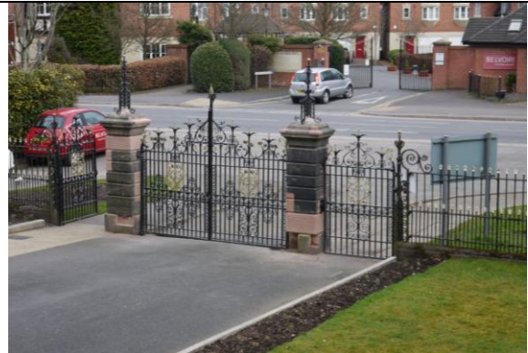
39. Restored gates and gate piers
