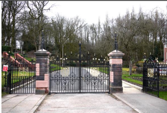
38. Restored gates and gate piers
