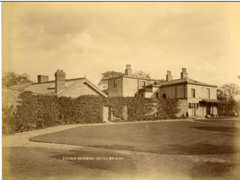
7. Winnington Bank House, now Victoria Infirmary
